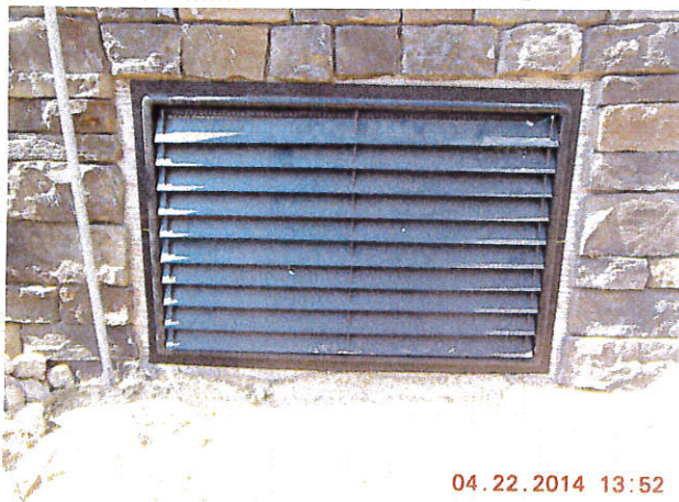
CRAWL SPACE DOOR VENT - TYPICAL OF 2
